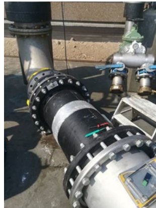
Figure 3-2 Antenna mounted on the fish factory pumping system
