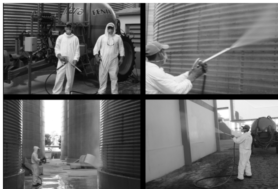
Figure 2 Buildings and silo sanitation. Prior grain filling silos were washed with pressurized water and a mixture of diatomaceous earth + deltamethrin was applied on the outside walls of buildings and silos.
